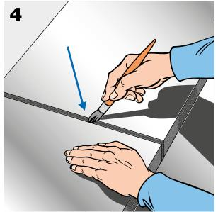
Mark the measurements of the surface to be insulated on the sheeting and cut the required size out of the roll.
